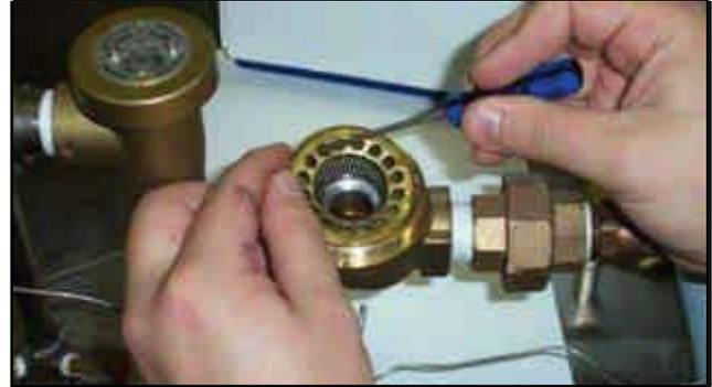
Removing the screen retainer
