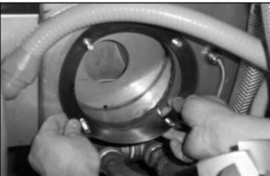
Removing the pump gasket
